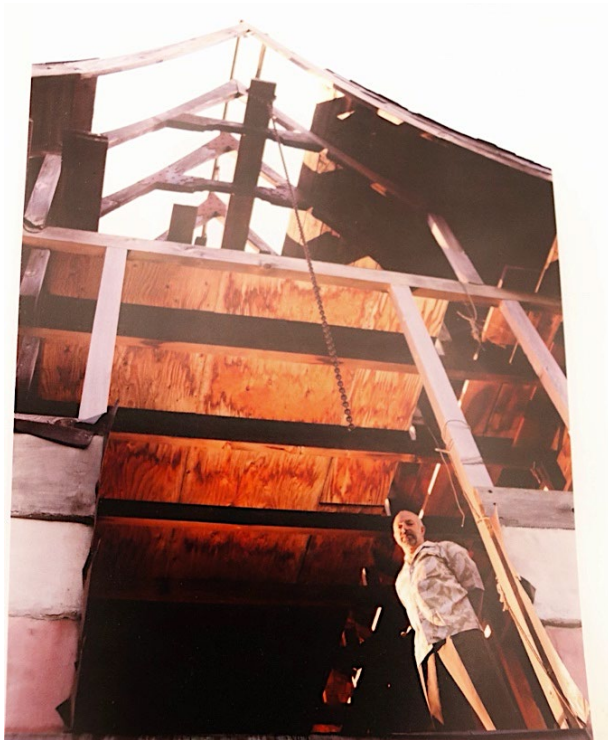
Figure 13. David Lee Hoffman with Teahouse under construction c. 1987.
