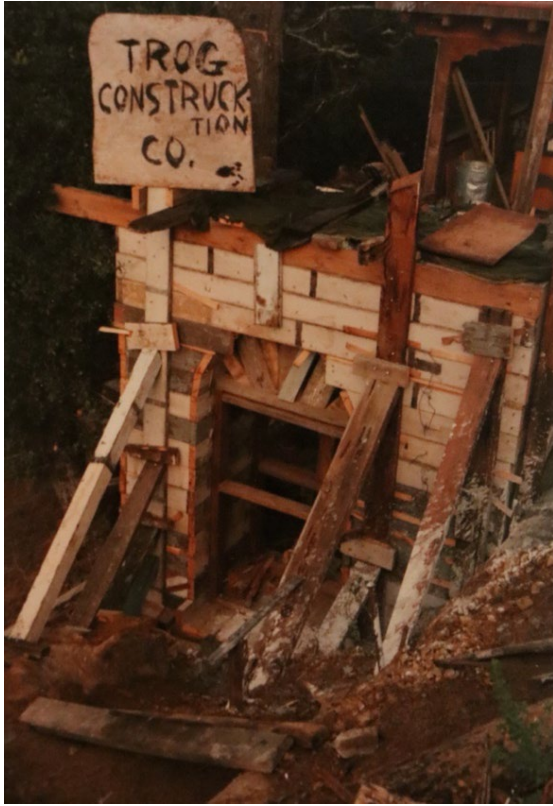
Figure 12. Woodshed Addition under construction, c. 1984. Photo Courtesy Susan Shannon.
